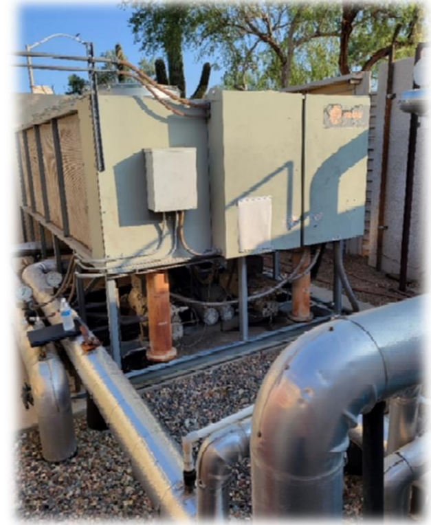
Existing 80 ton chiller with two 40 ton compressors
