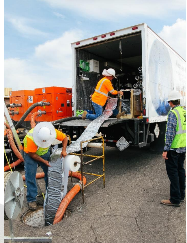
Liner Installation
