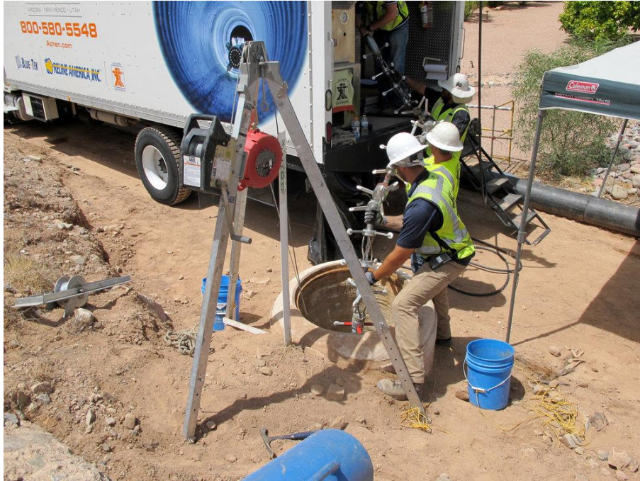
UV Light Installation
