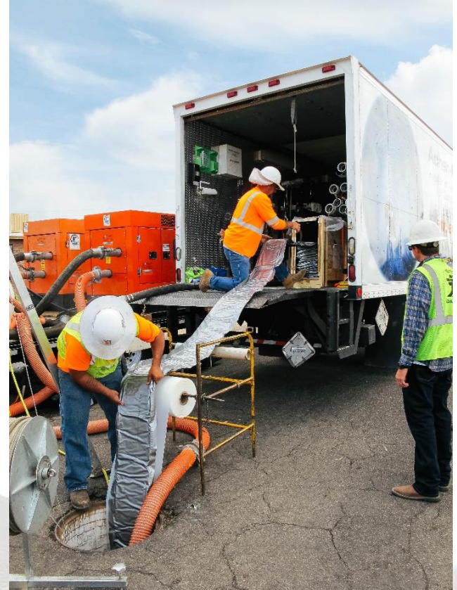
Liner Installation
