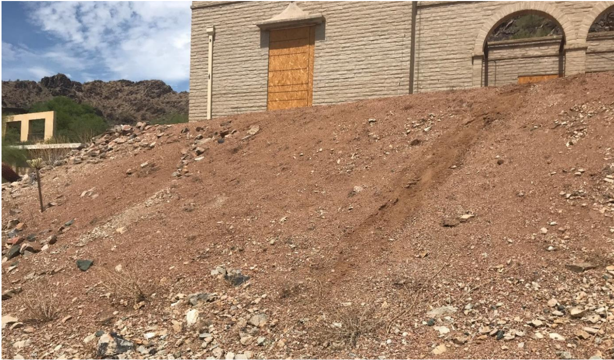
Figure 5: General site conditions showing the existing residential structure and fill slope – although that it appears that the fill may be 10 to 12 feet, the buried natural slope beneath supports that the actual fill thickness reaches a maximum of 8.0 feet
