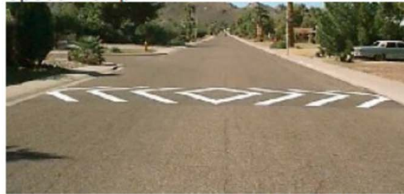
Figure 2-24 Speed Humps
