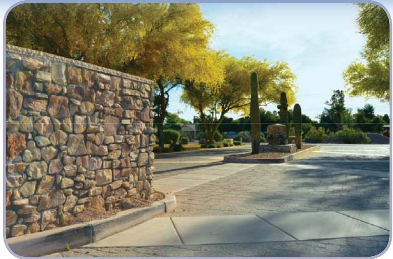
*Figure 7: Existing Use of Stone Veneer, Rustic Pavers, and Concrete.*
