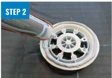
APPLY CHEMLINK M1 SEALANT
