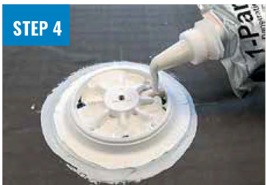
FILL WITH CHEMLINK 1-PART & PLACE CAP
