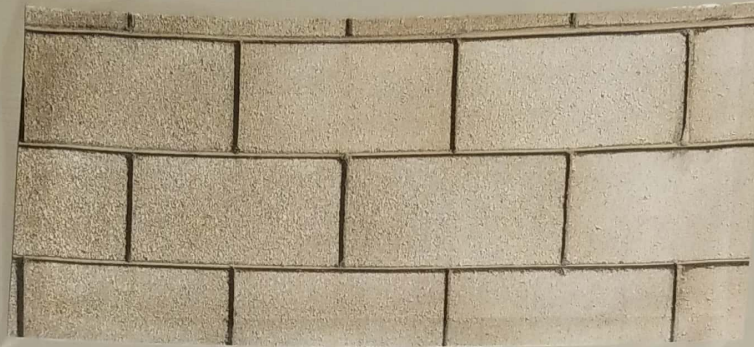
Accent walls – exposed CMU block with black mortar
