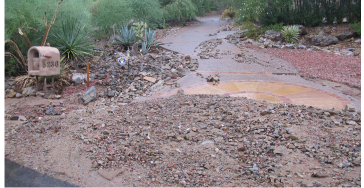
Erosion in Paradise Valley
