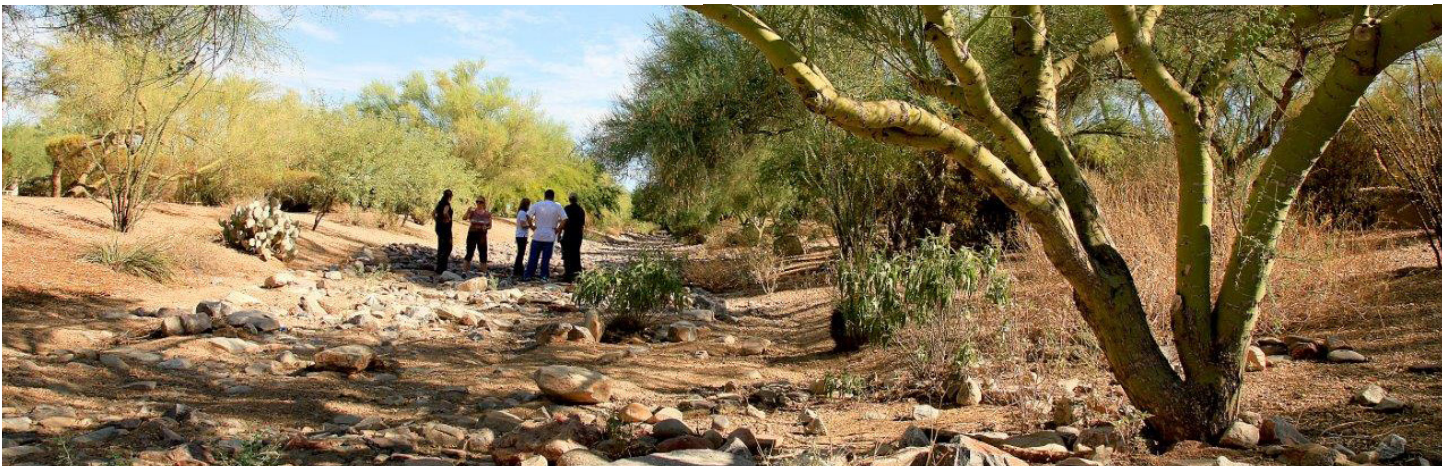
Stormwater management facilities integrated with natural landscape
