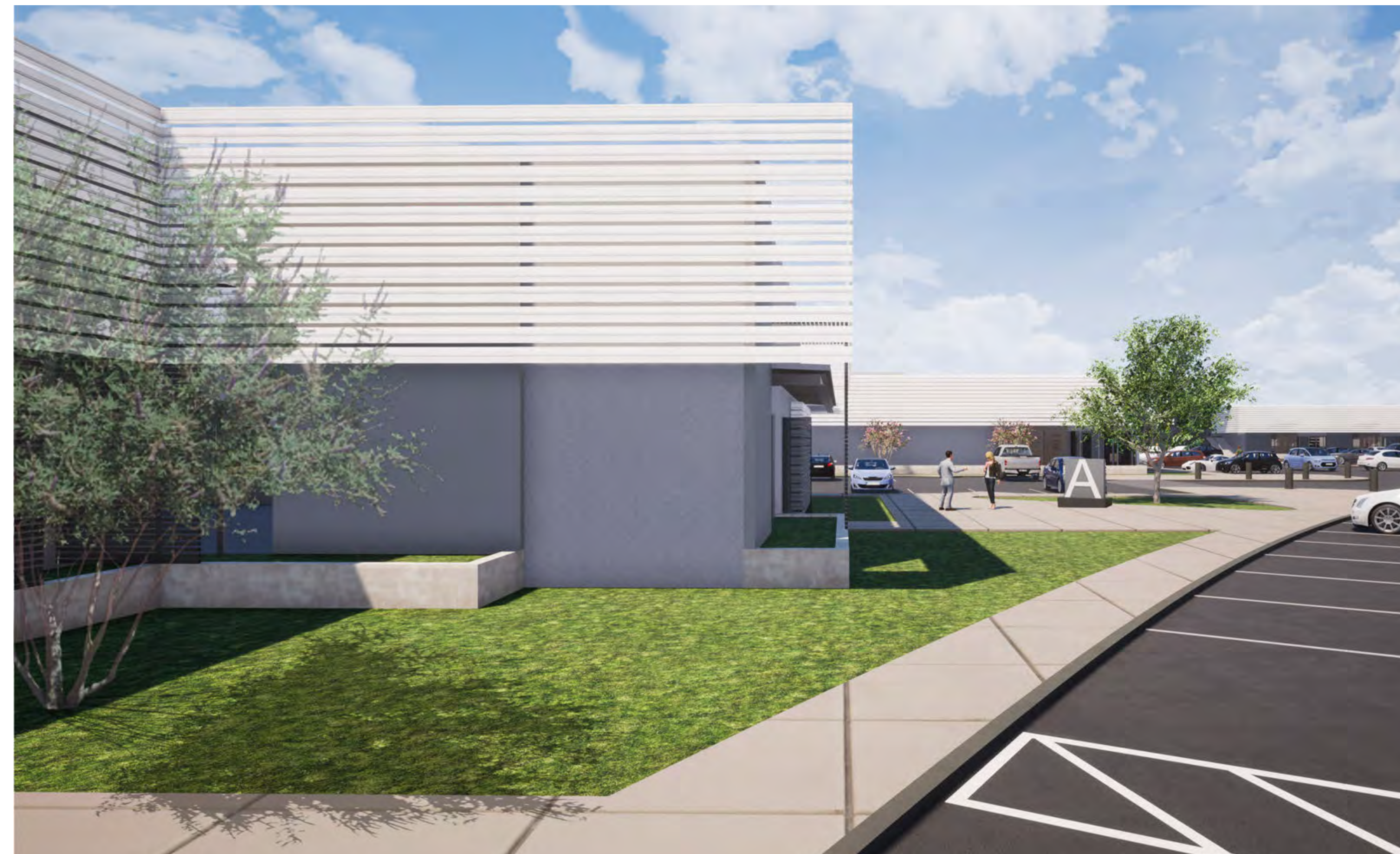
VIEW OF BLDG A LOOKING NORTH
