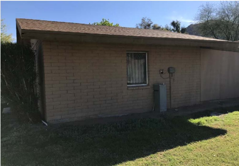
Figure 2 Existing Shed - North Elevation - Looking Southwest
