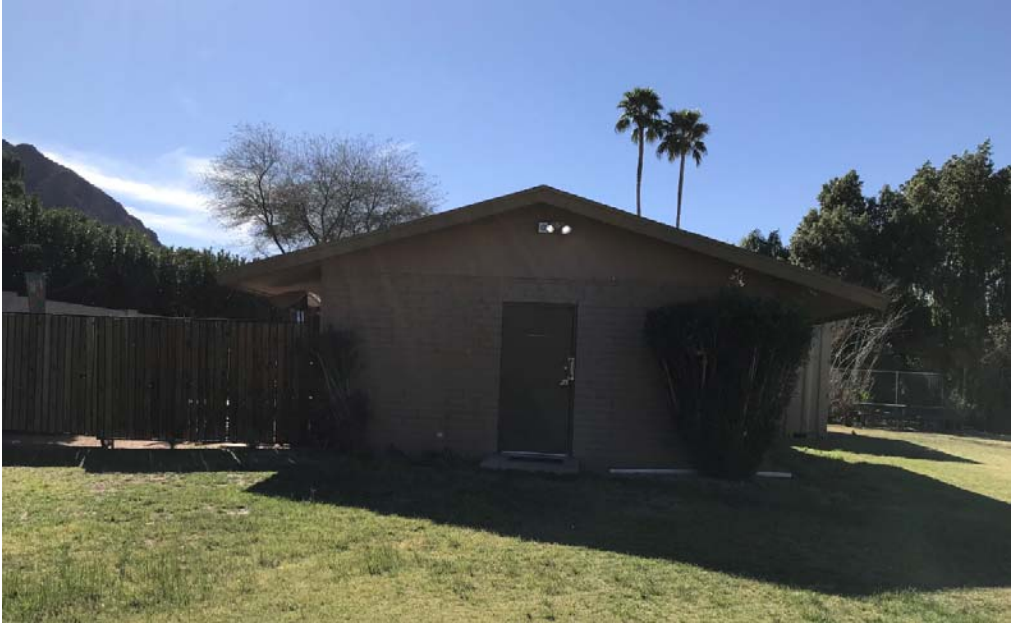
Figure 1 Existing Shed - East Elevation - Looking West
