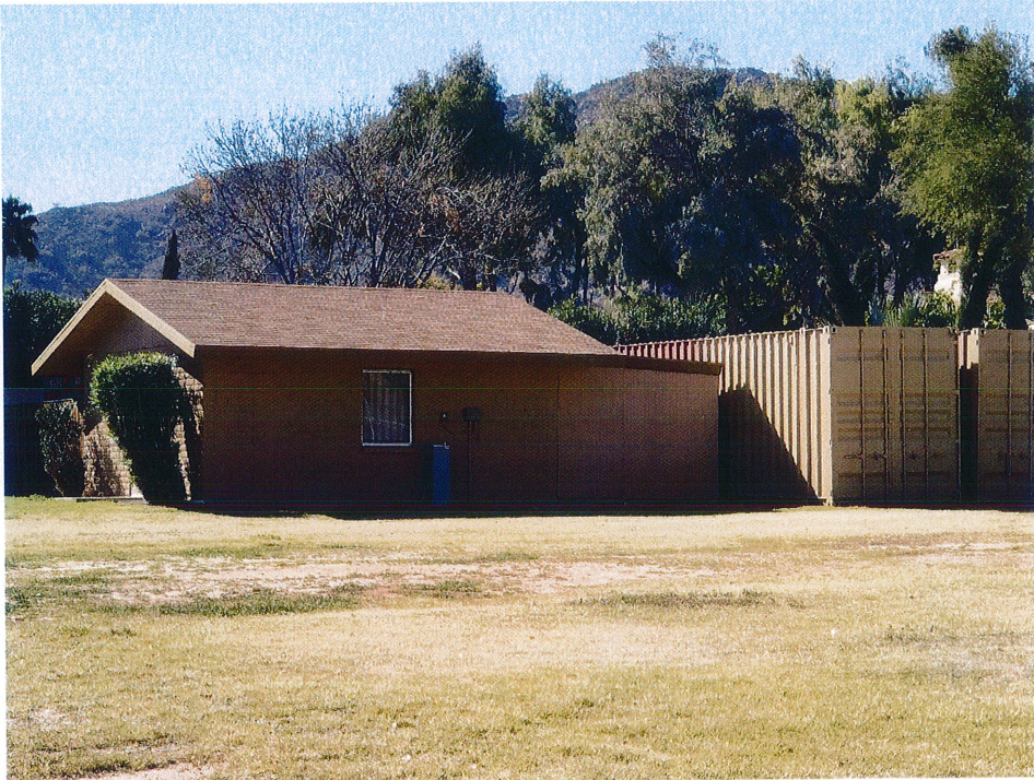
Maintenance Building with painted pods
