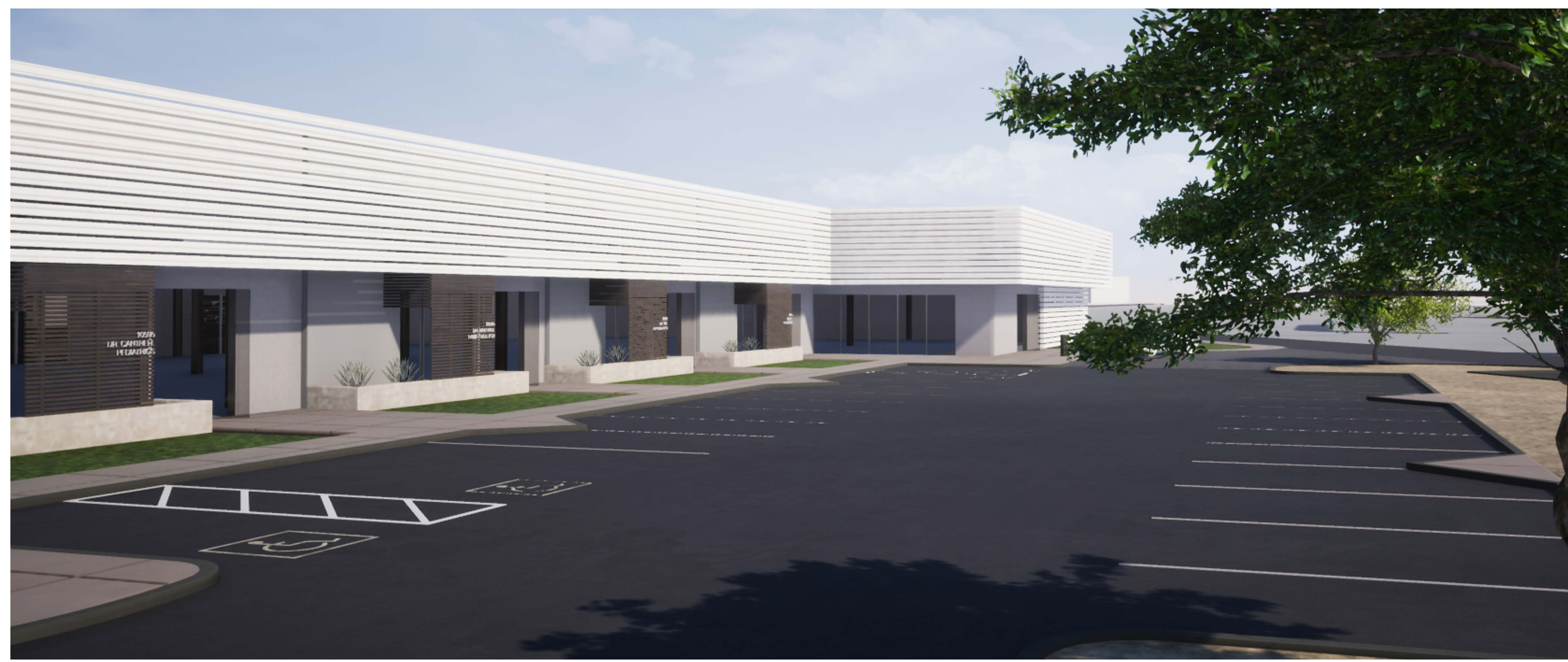
VIEW OF BUILDING F
