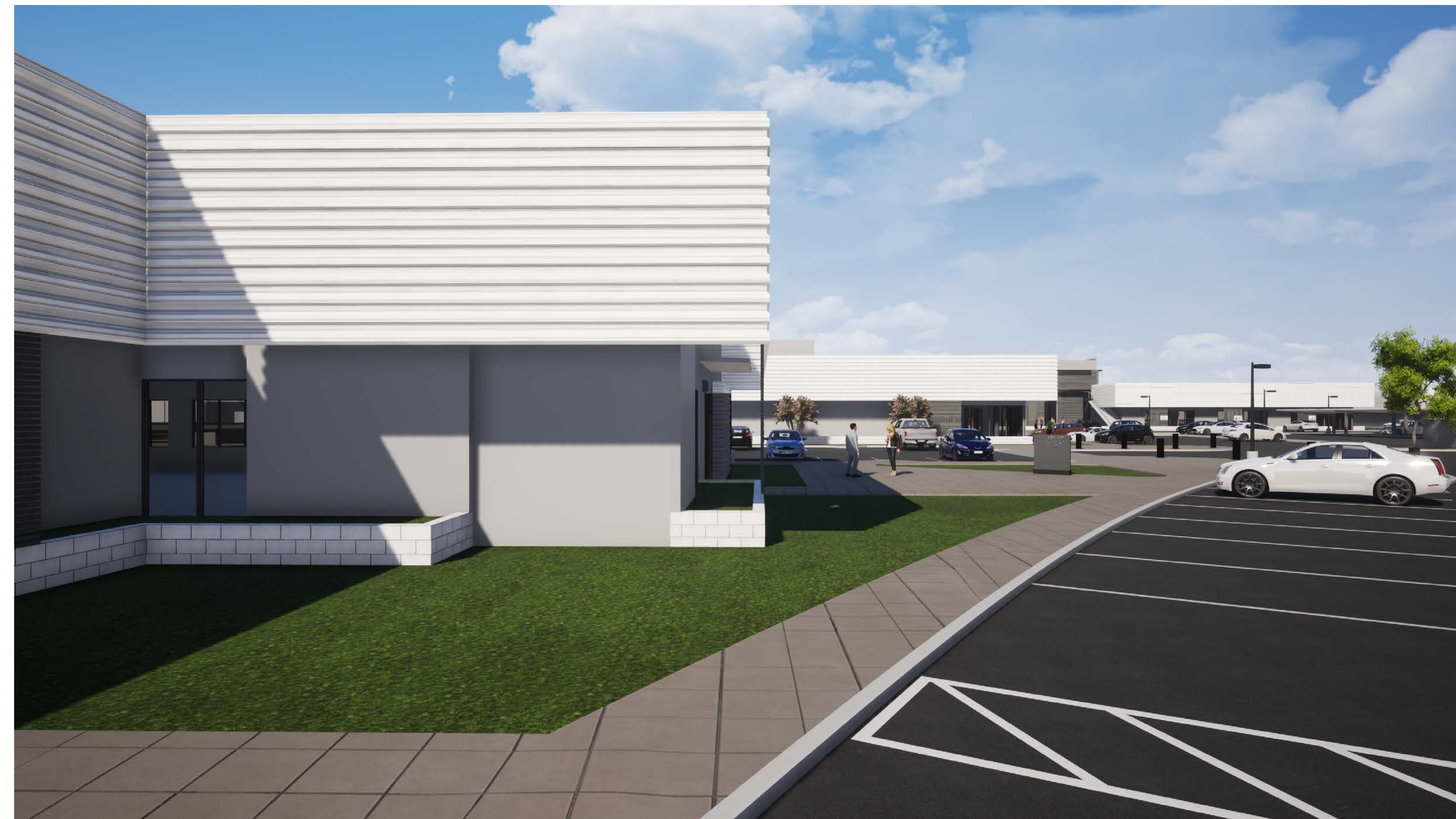
VIEW OF BLDG A LOOKING NORTH
