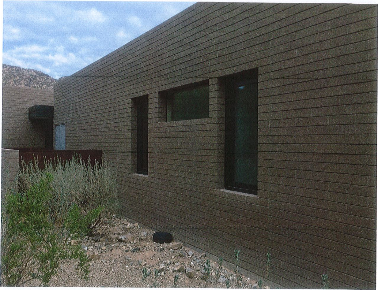
Rear Elevation SE Corner
