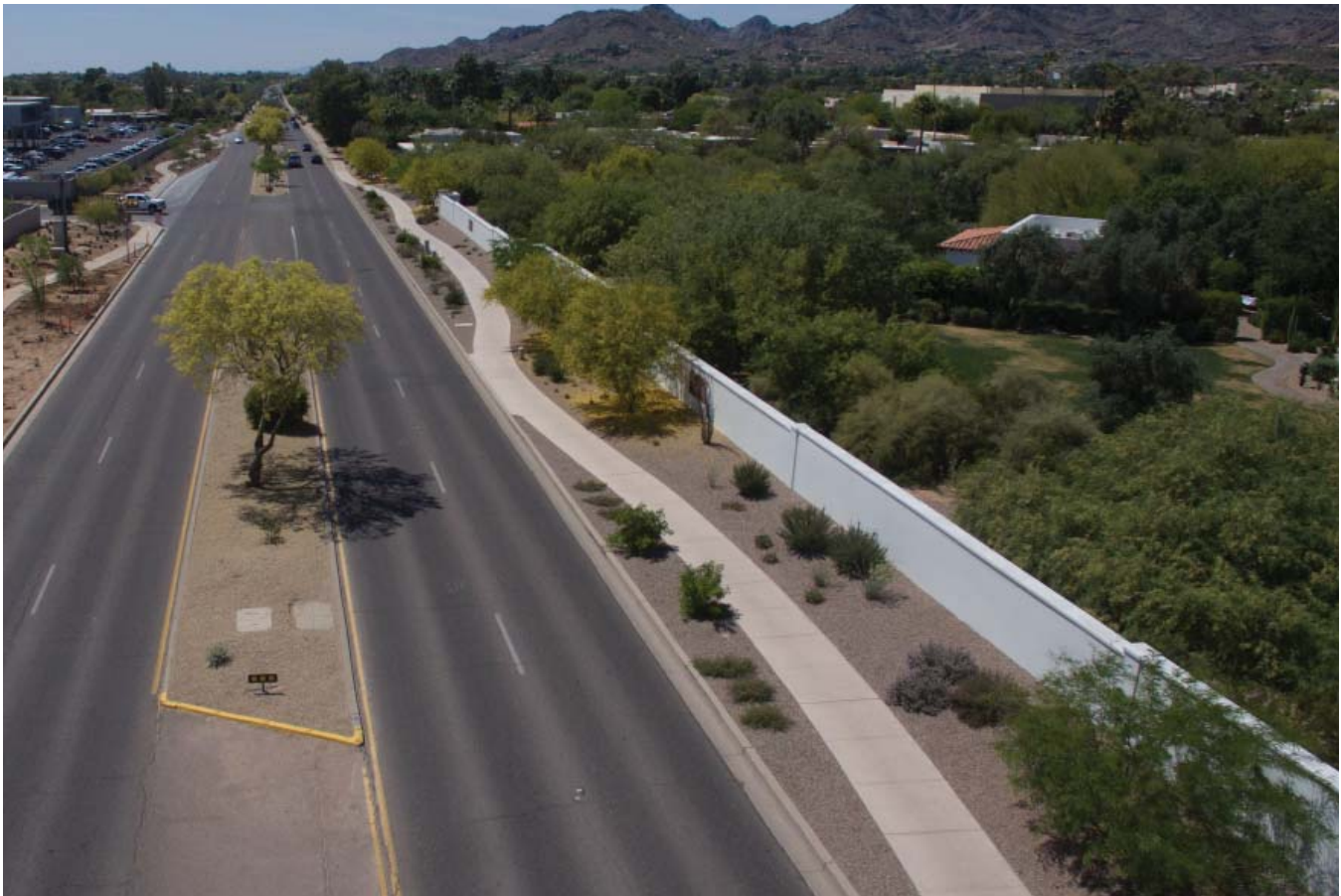
Figure 4.1: Landscape, Sidewalk and Oleander Hedge Replacement Improvements on Lincoln Drive Completed in 2015
