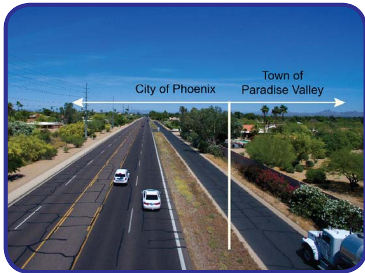
Figure 3.3: Tatum Boulevard Looking North, Demonstrating Right-of-Way Limitations
