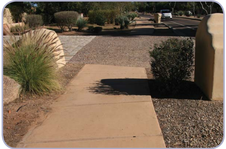
Figure 2.7: Existing Use of Colored Concrete, Exposed Aggregate, and Rustic Pavers
