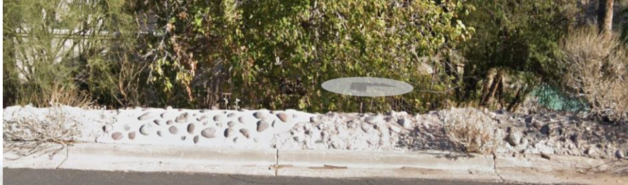
Existing Grouted Rip-Rap
