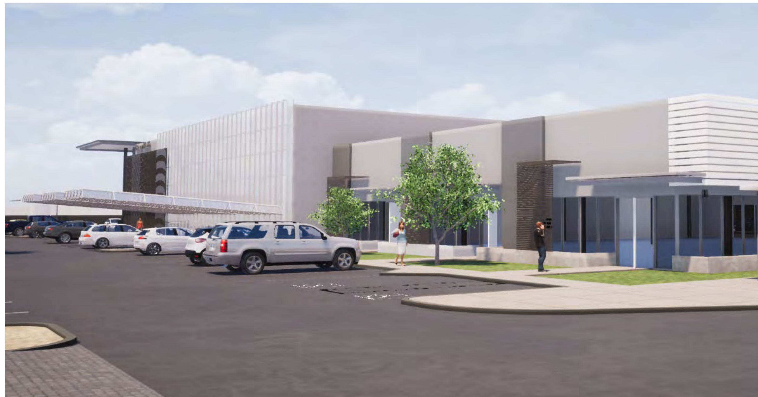
VIEW OF BUILDING A ENTRIES
