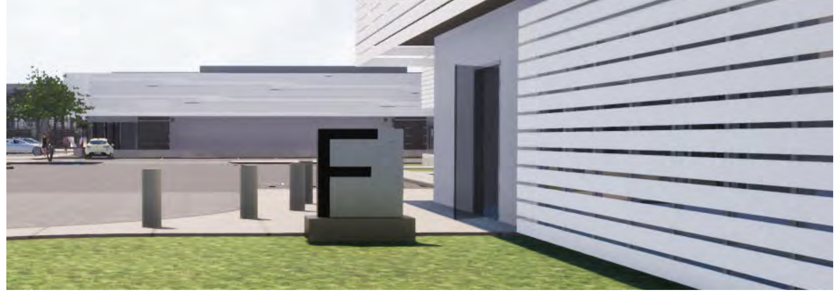
SIGN NO. 6 AT BLDG F
