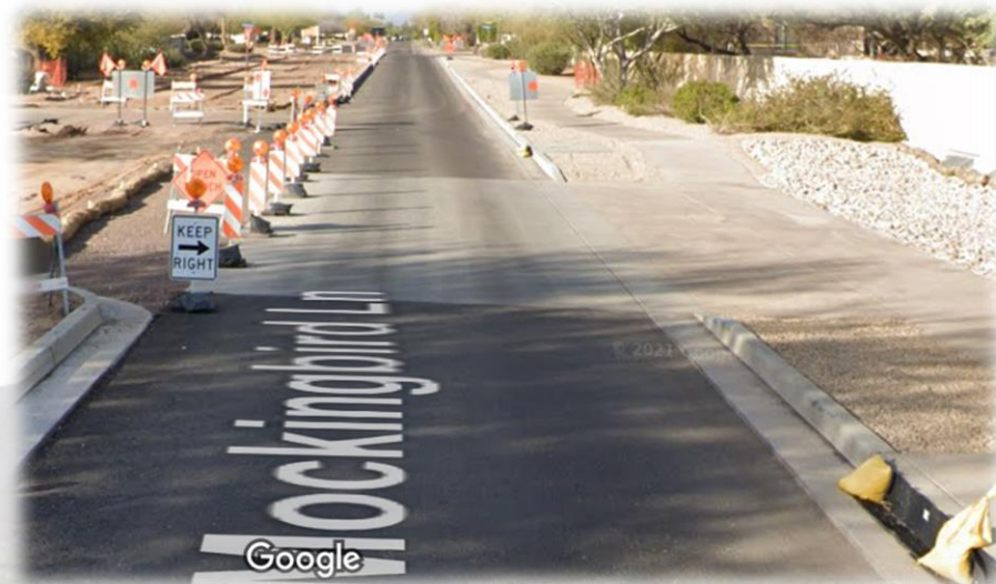
Concrete Crossing (north of Indian Bend Rd)
