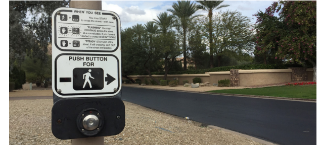
Figure 2-28 Crossing Pedestrian Button/Bike Sensor
