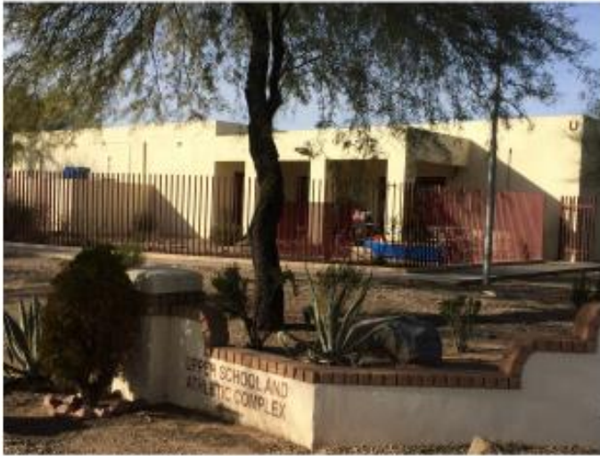
1 ARTS & SCIENCES BUILDING COURTYARD FENCE "BEFORE"
