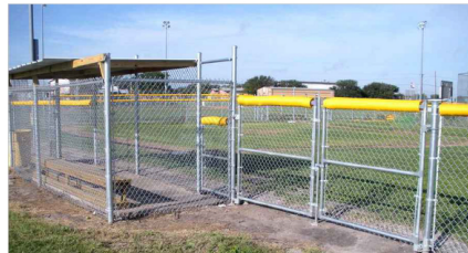
BASEBALL FIELD CHAIN LINK FENCE EXHIBIT
