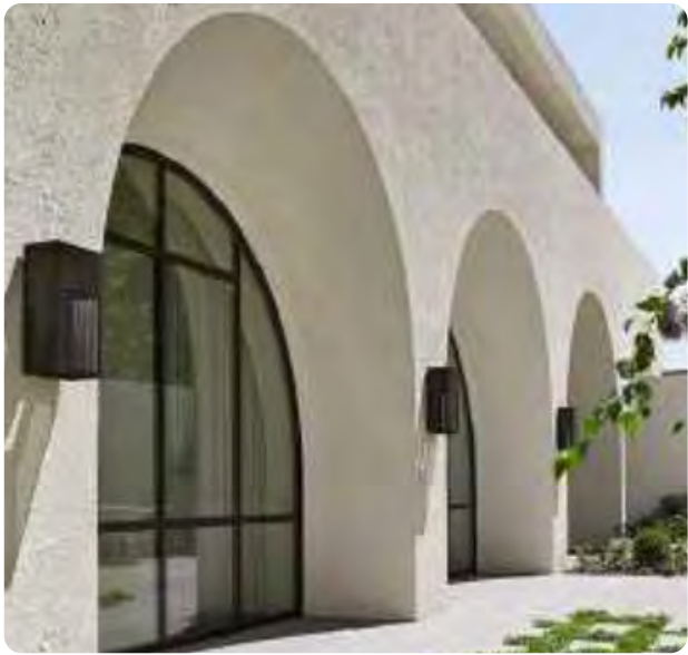
NEW ENTRY DOORS
