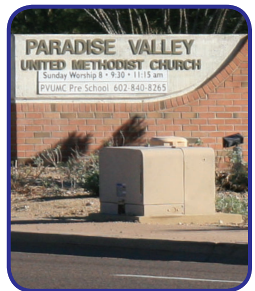
Figure 2.6: Existing Painted Utility
