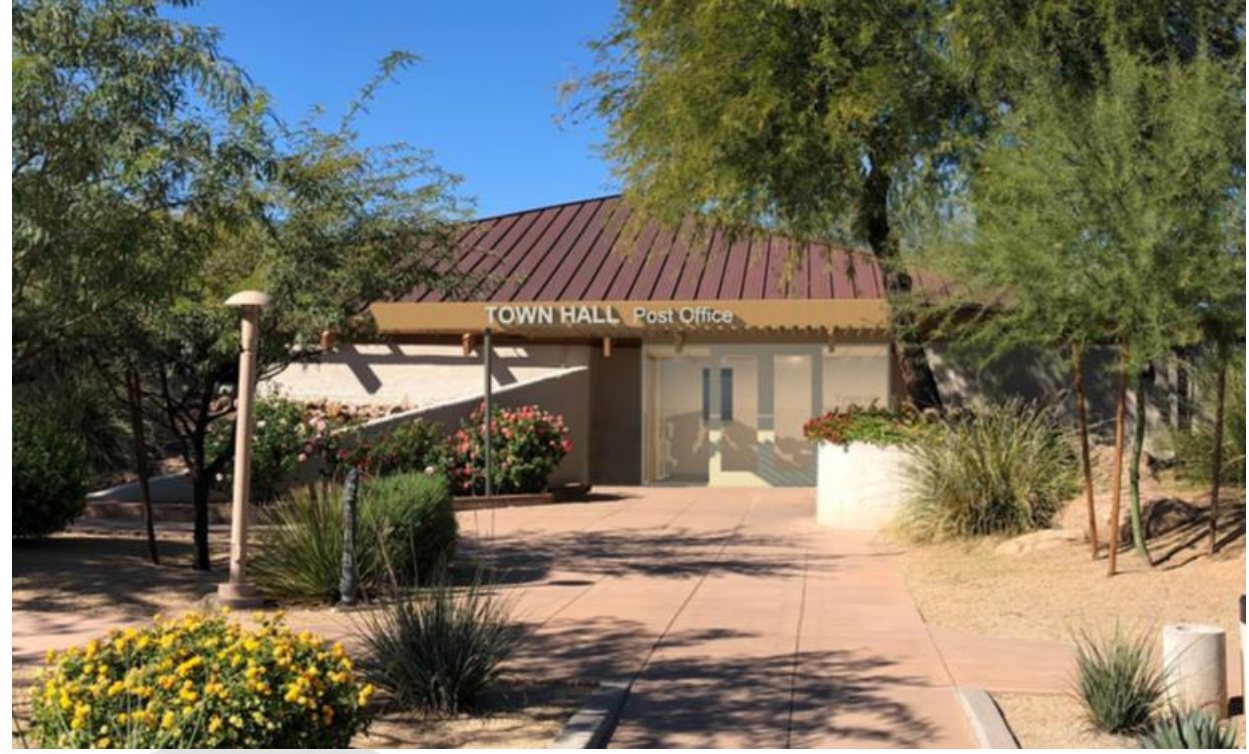
New front entry with shade canopy
