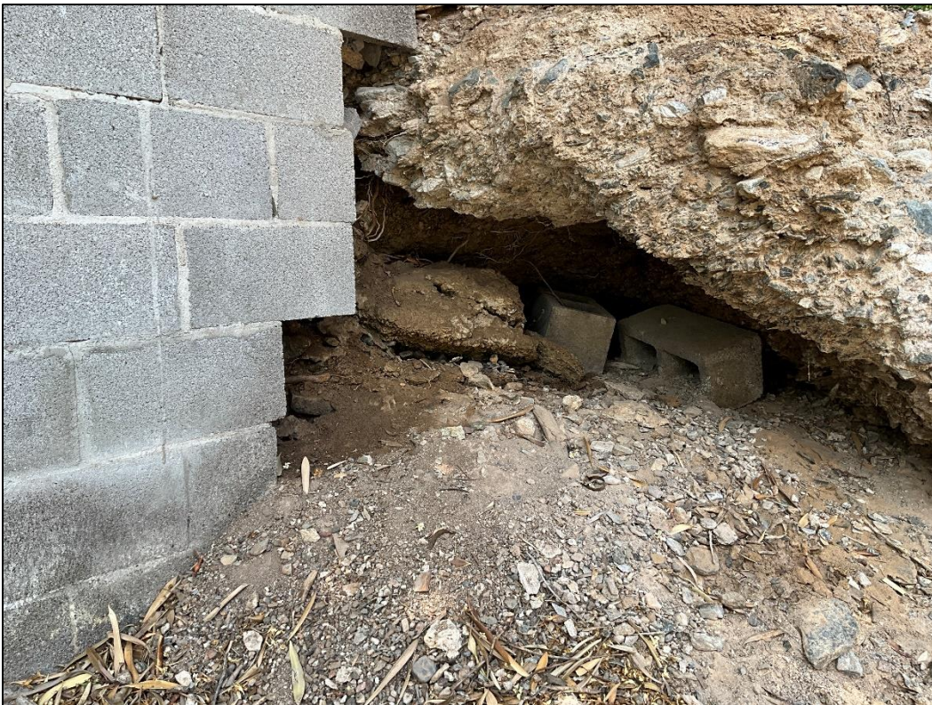
Figure 4: Current site conditions – fanglomerate undercutting
