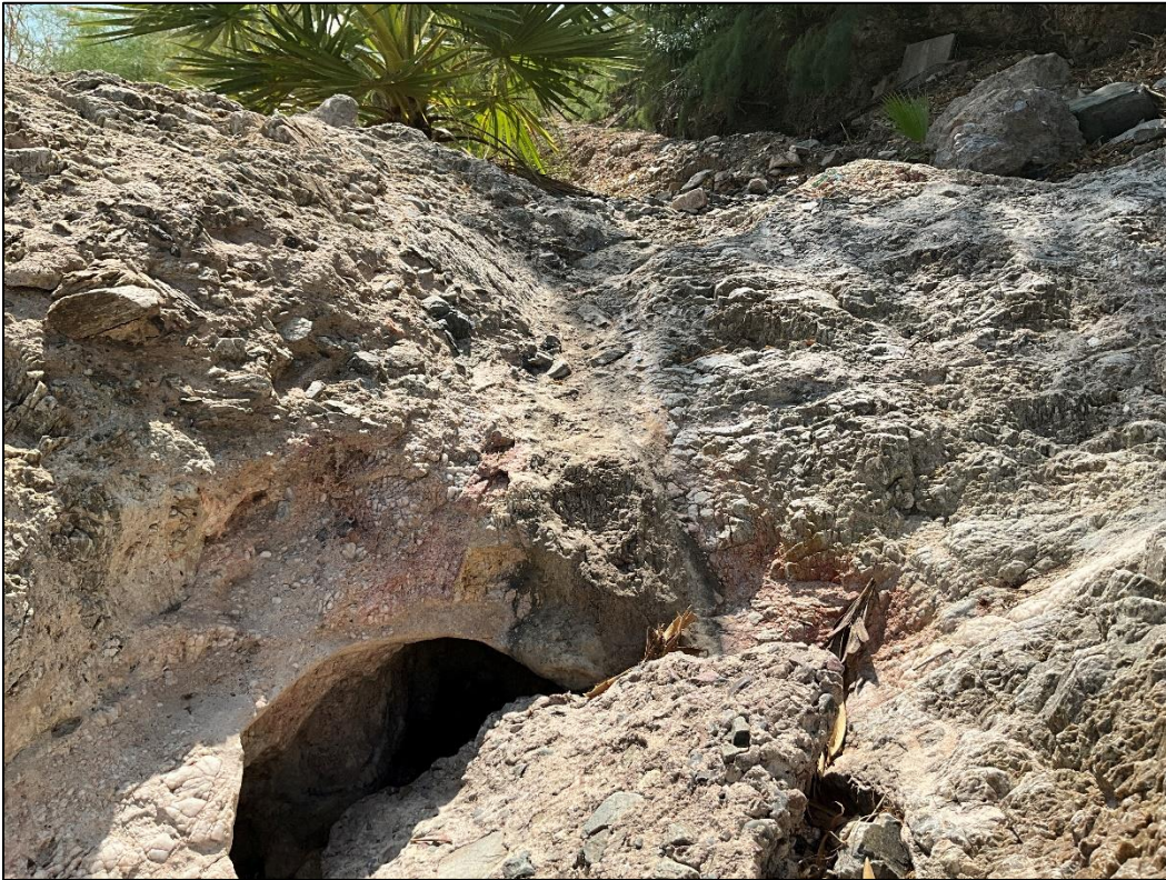
Figure 5: Current site conditions – fanglomerate undercutting
