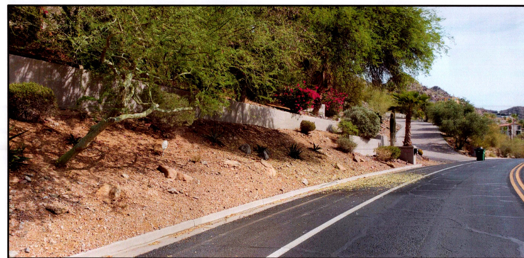
6 EXISTING SITE PICTURE
