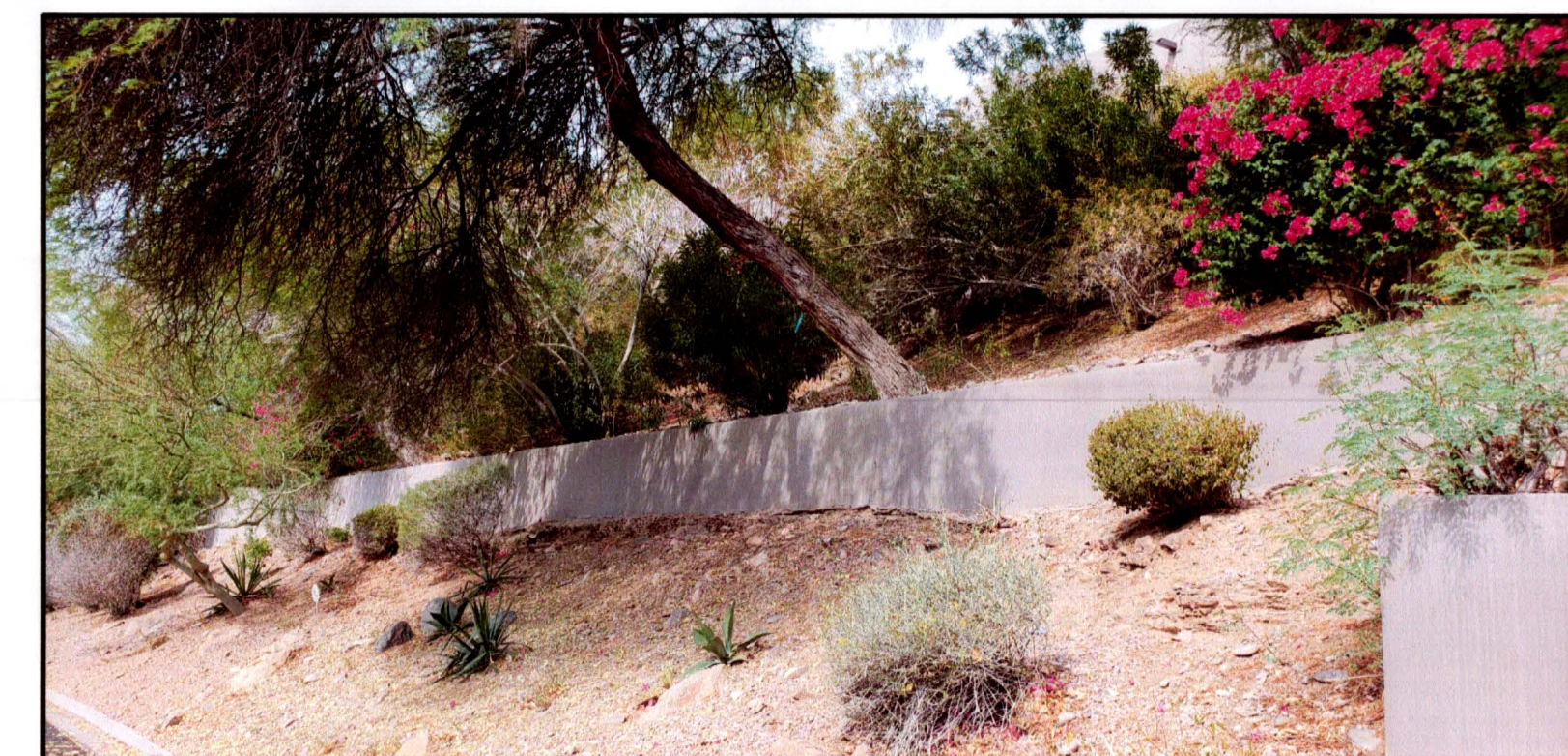
4 EXISTING SITE PICTURE
