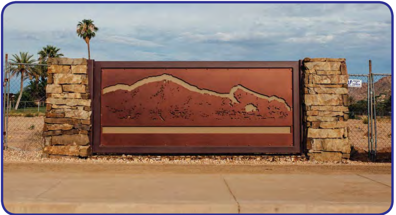
Figure 2.13: Existing Utility Screens at 56th Street, South of Lincoln
