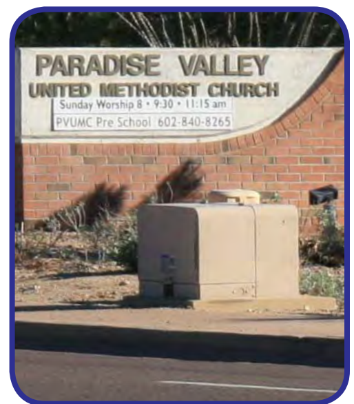
Figure 2.10: Existing Painted Utility
