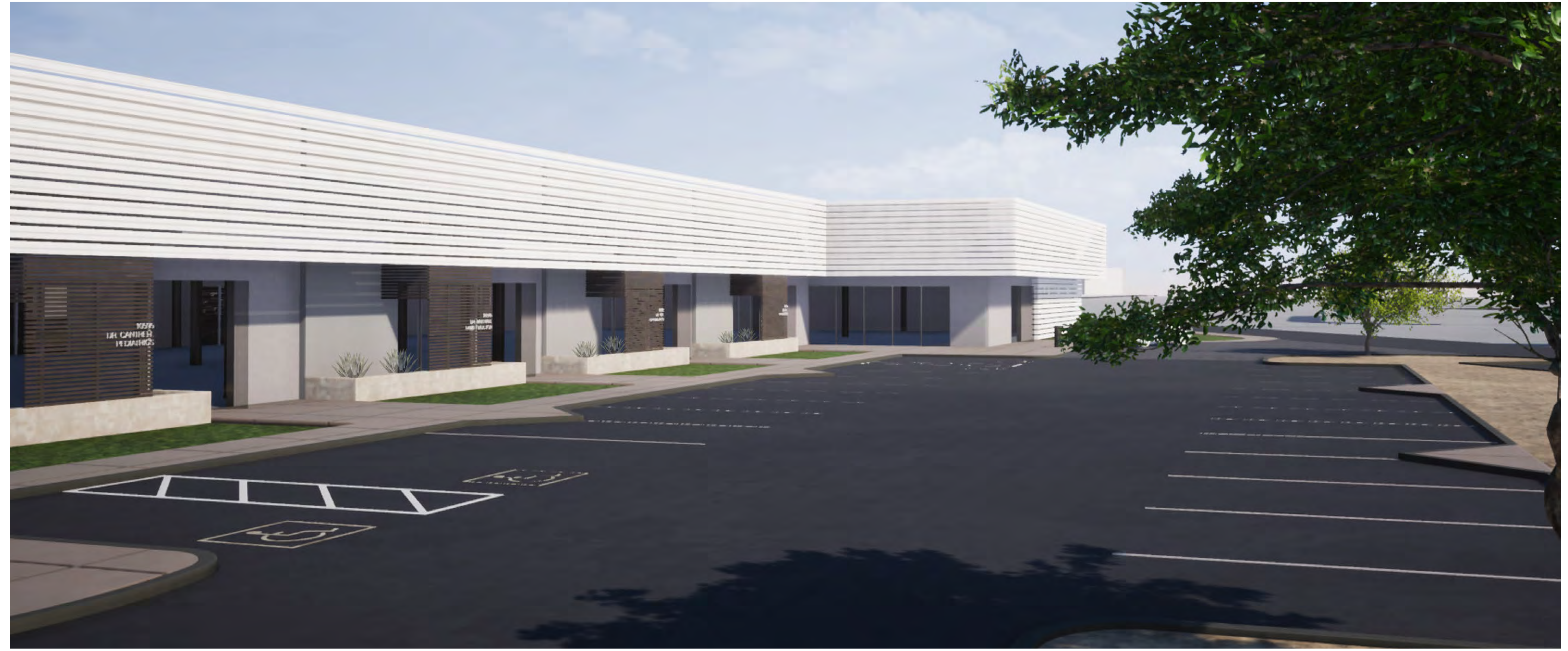
VIEW OF BUILDING F
