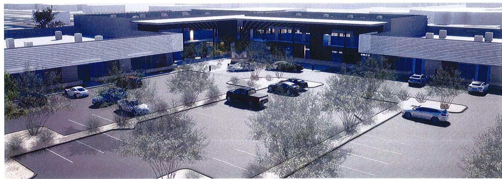
BLDGS B,C,D,E LOOKING NORTH WEST
