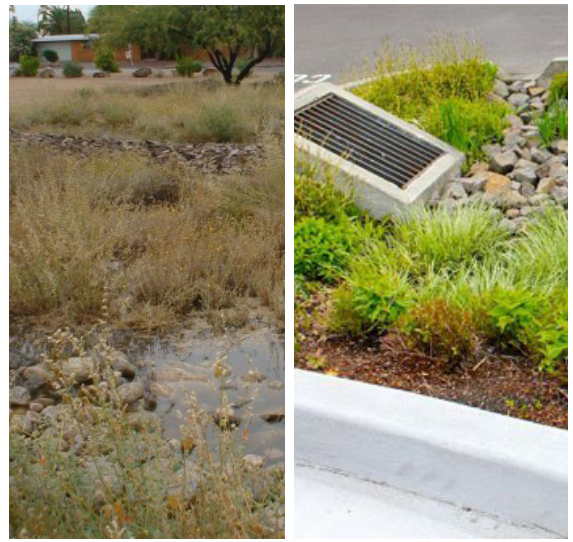
Bioretention areas detain stormwater while enhancing the landscape.
