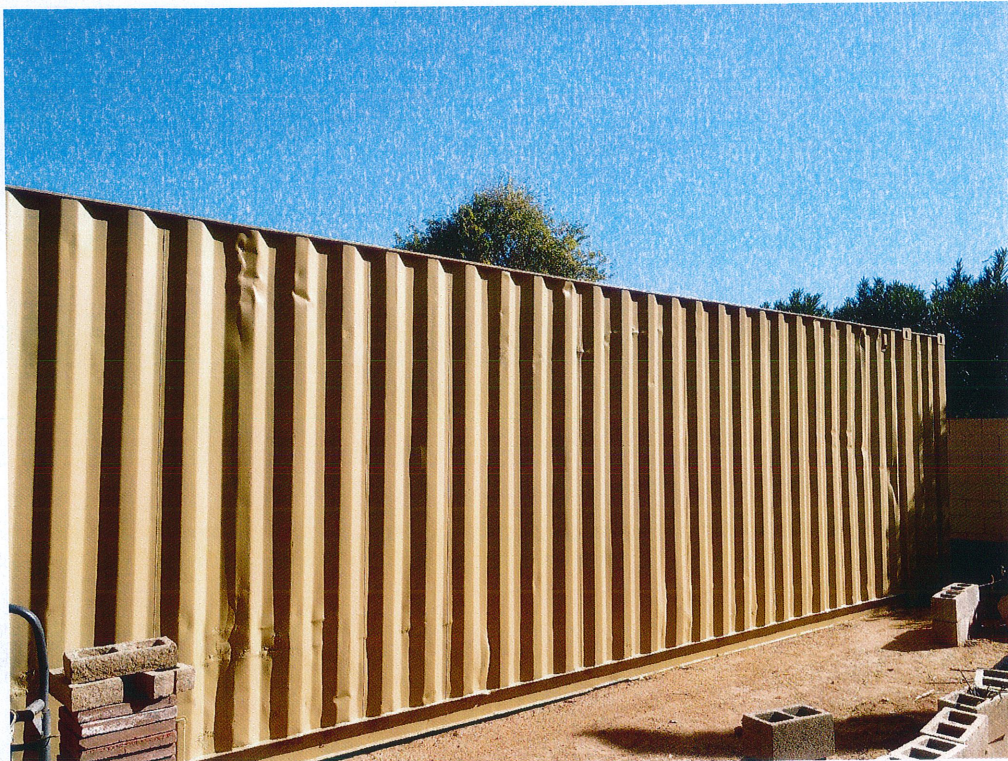
Painted Pod – similar to a wall
