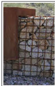
Sample gabion wall- rock type tbd
