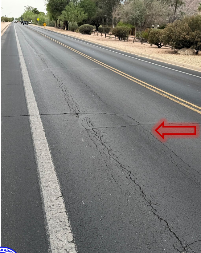
Utility trench settling
