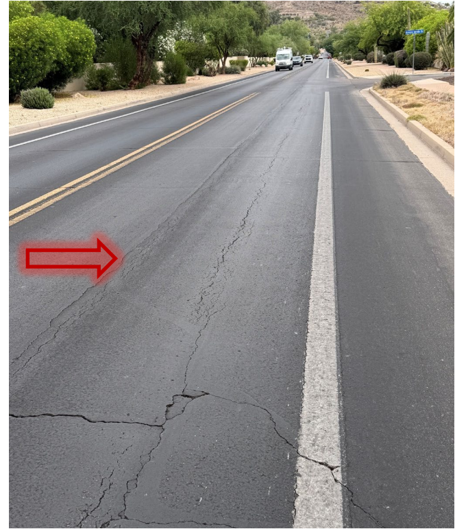
Utility trench settling
