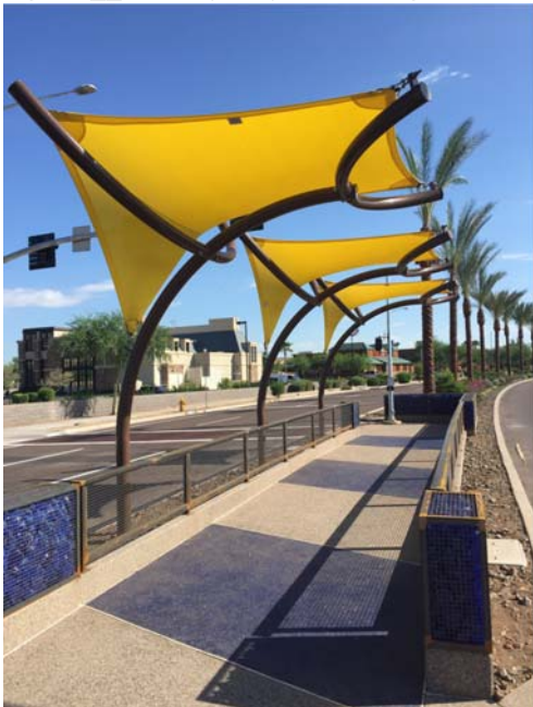
Figure __: Example of Z-Crossing with a shaded pedestrian refuge within center median. (photo J2 Design)
