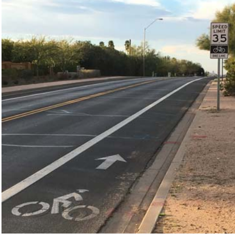
Figure __: Existing Pavement Markings in Paradise Valley
