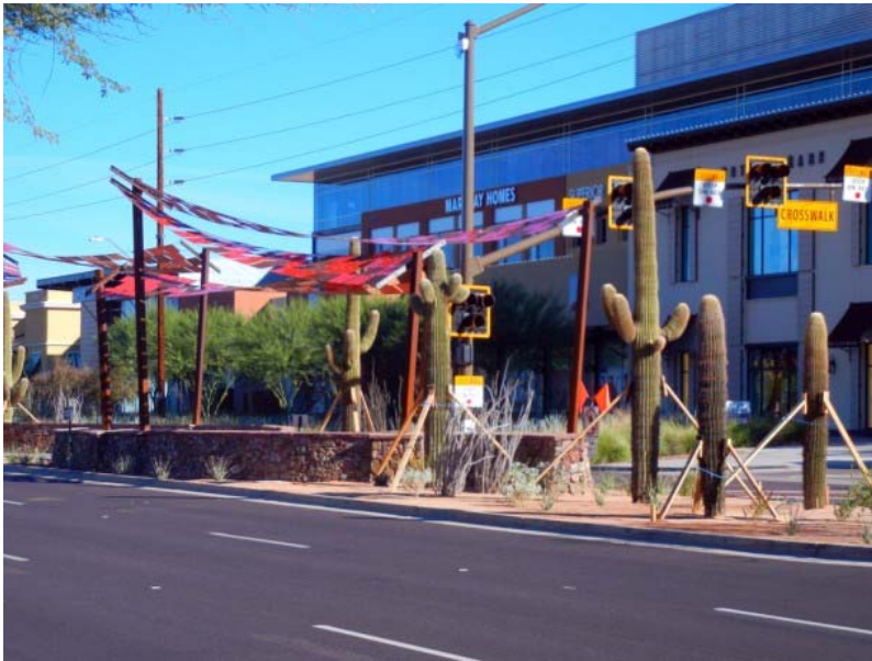
Figure __: Example of a HAWK Beacon and Z-Crossing with Enhanced Crosswalk Paving at Kierland/Scottsdale Quarter across Scottsdale Road. (photo Valley Rain)
