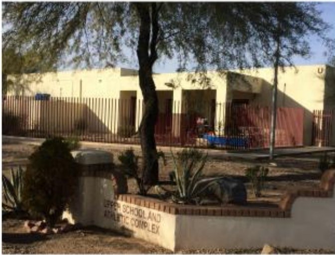
1 ARTS & SCIENCES BUILDING COURTYARD FENCE "BEFORE"
