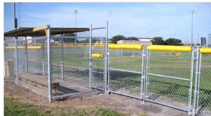
BASEBALL FIELD CHAIN LINK FENCE EXHIBIT
