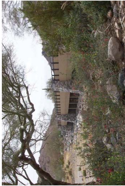
Example of Box Culvert Bridge. Wash Crossing In Parcel B to be Similar In Design.
