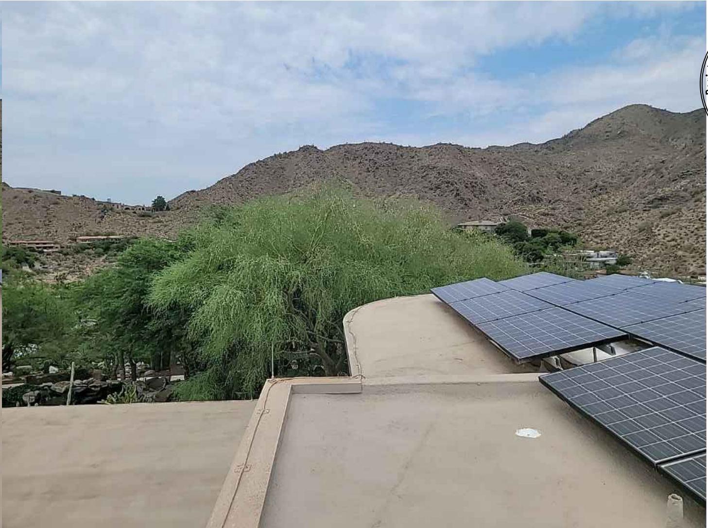
PARAPET WALL #4 (PARAPET HEIGHT (EST.): 6")
