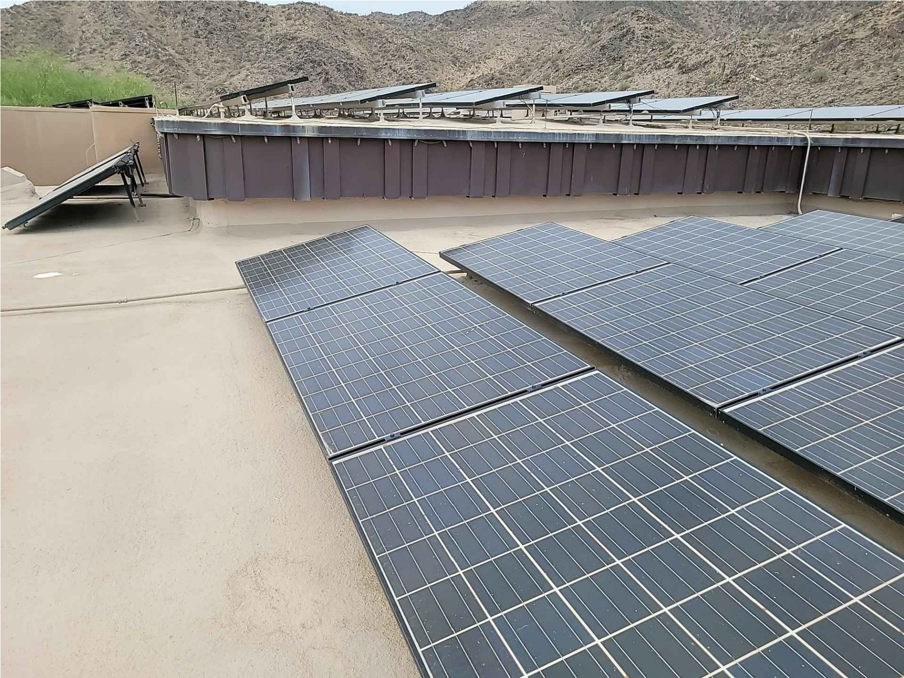
PARAPET WALL #1 (PARAPET HEIGHT: 3'-9")
