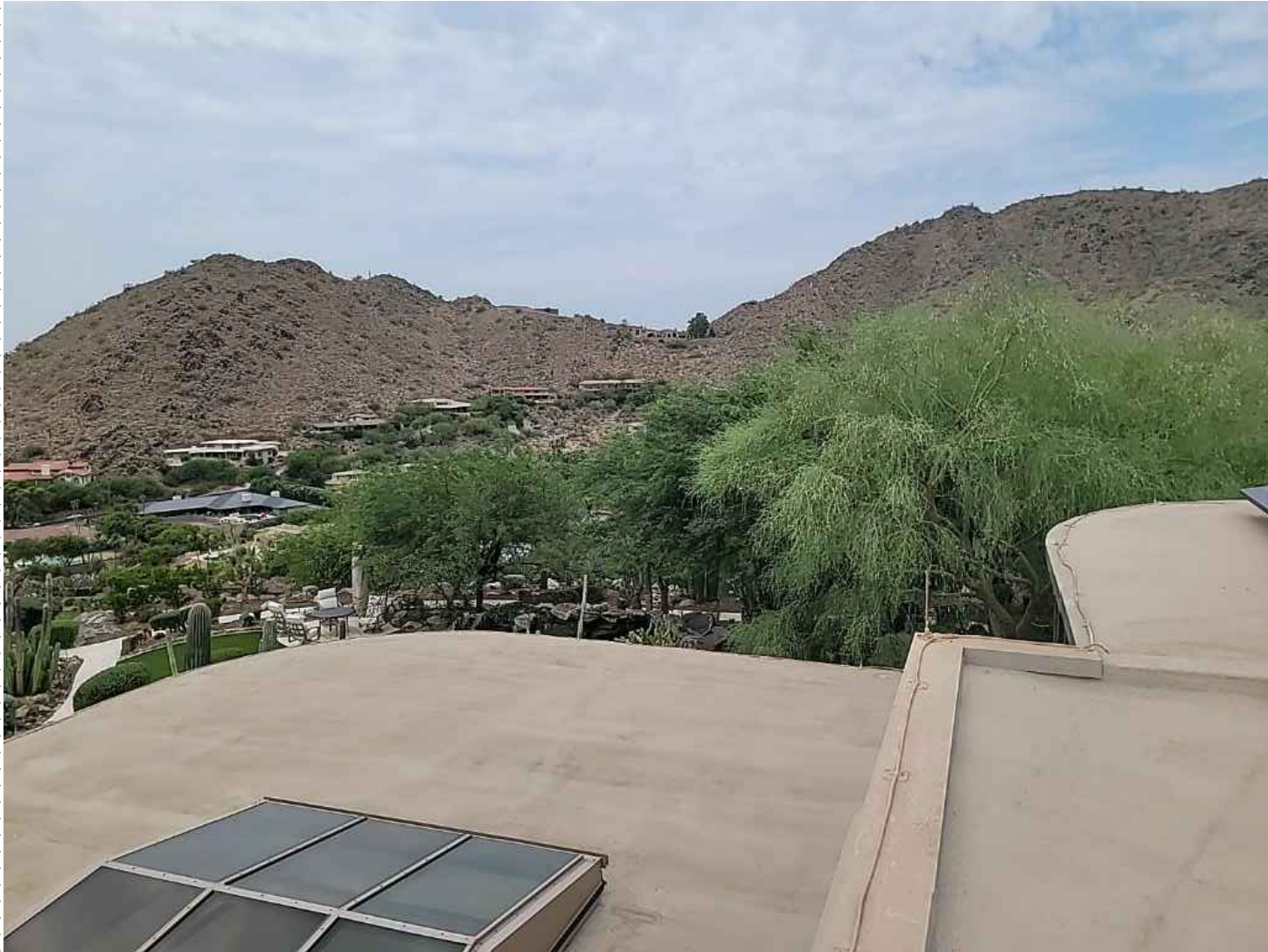
PARAPET WALL #3 (PARAPET HEIGHT (EST.): 6")
