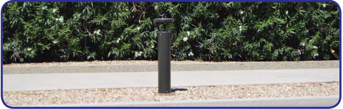
Figure 2.12: Solar Lighting Bollard
