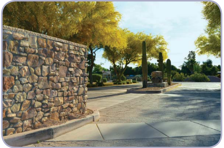
Figure 2.23: Example Use of Stone Veneer and Decorative Paving at Resort Setting
