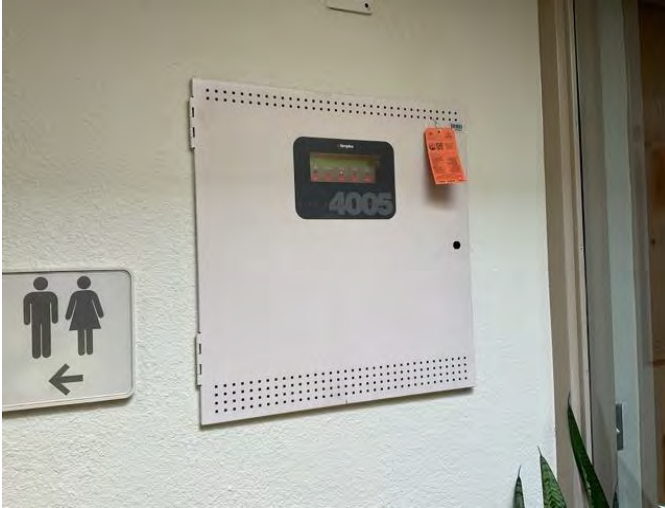
19 - NONCOMPLIANT FIRE ALARM PANEL
