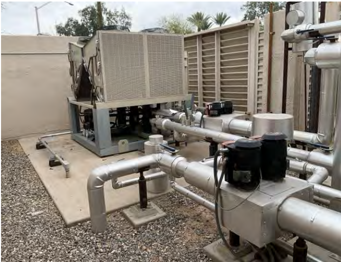
21 - AIR COOLED CHILLER AND PUMPS
