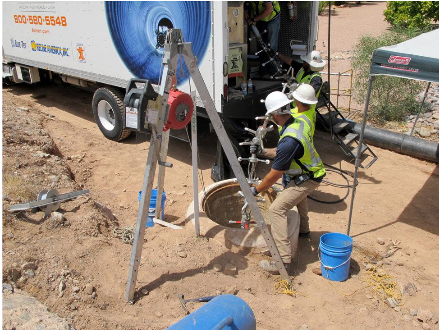
UV Light Installation
