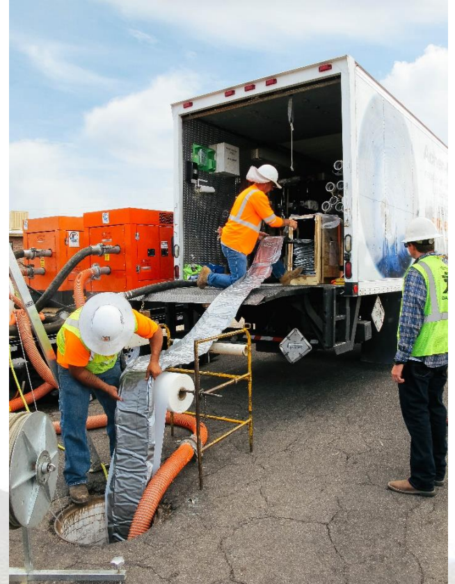
Liner Installation
