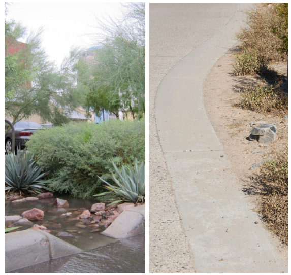
Curb cuts control stormwater flow from streets to LID facilities.
