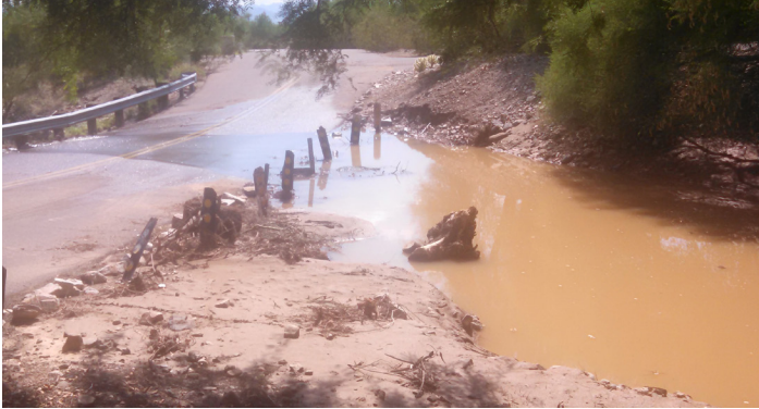
Fully charged drainage in Paradise Valley
