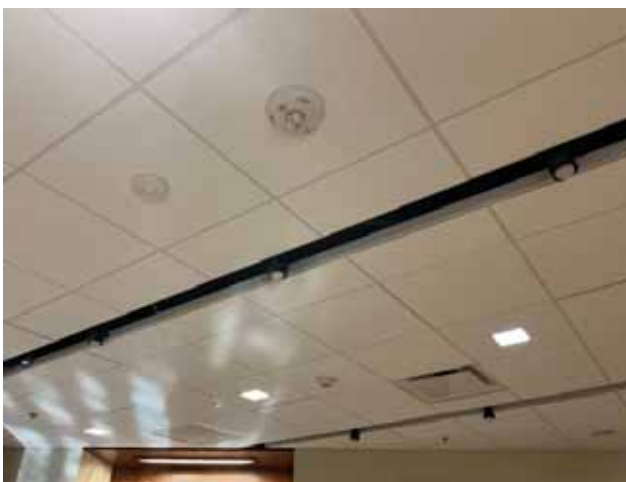
17 - FIRE ALARM COMPONENTS
