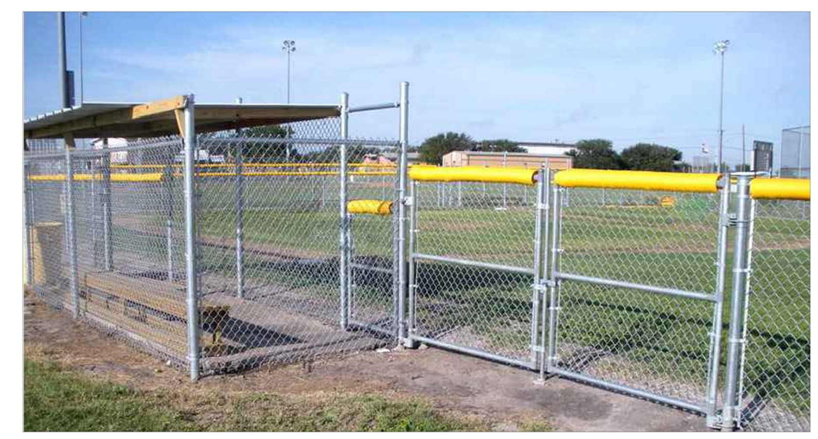
BASEBALL FIELD CHAIN LINK FENCE EXHIBIT
