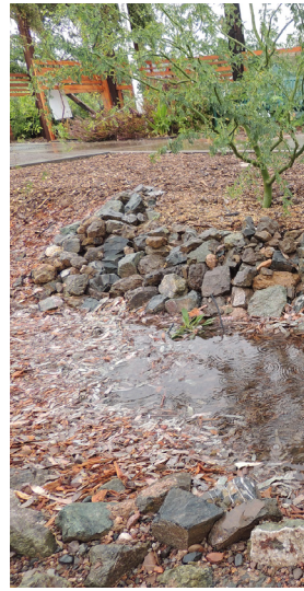
Vegetated swales accept stormwater for conveyance, storage and infiltration.
