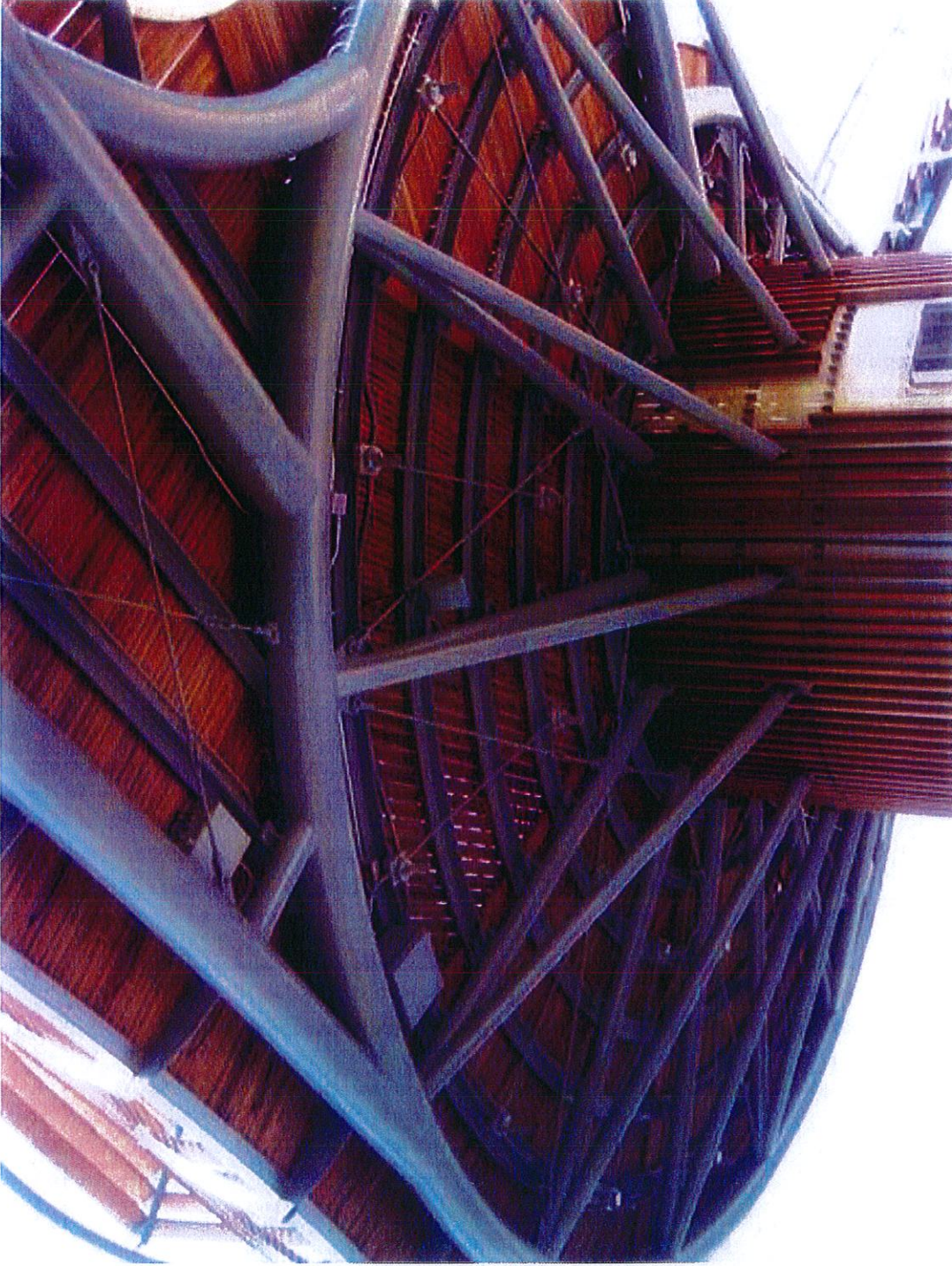
Figure 23. AT&T stealthed small facility deployment at Dallas Arboretum. 23
