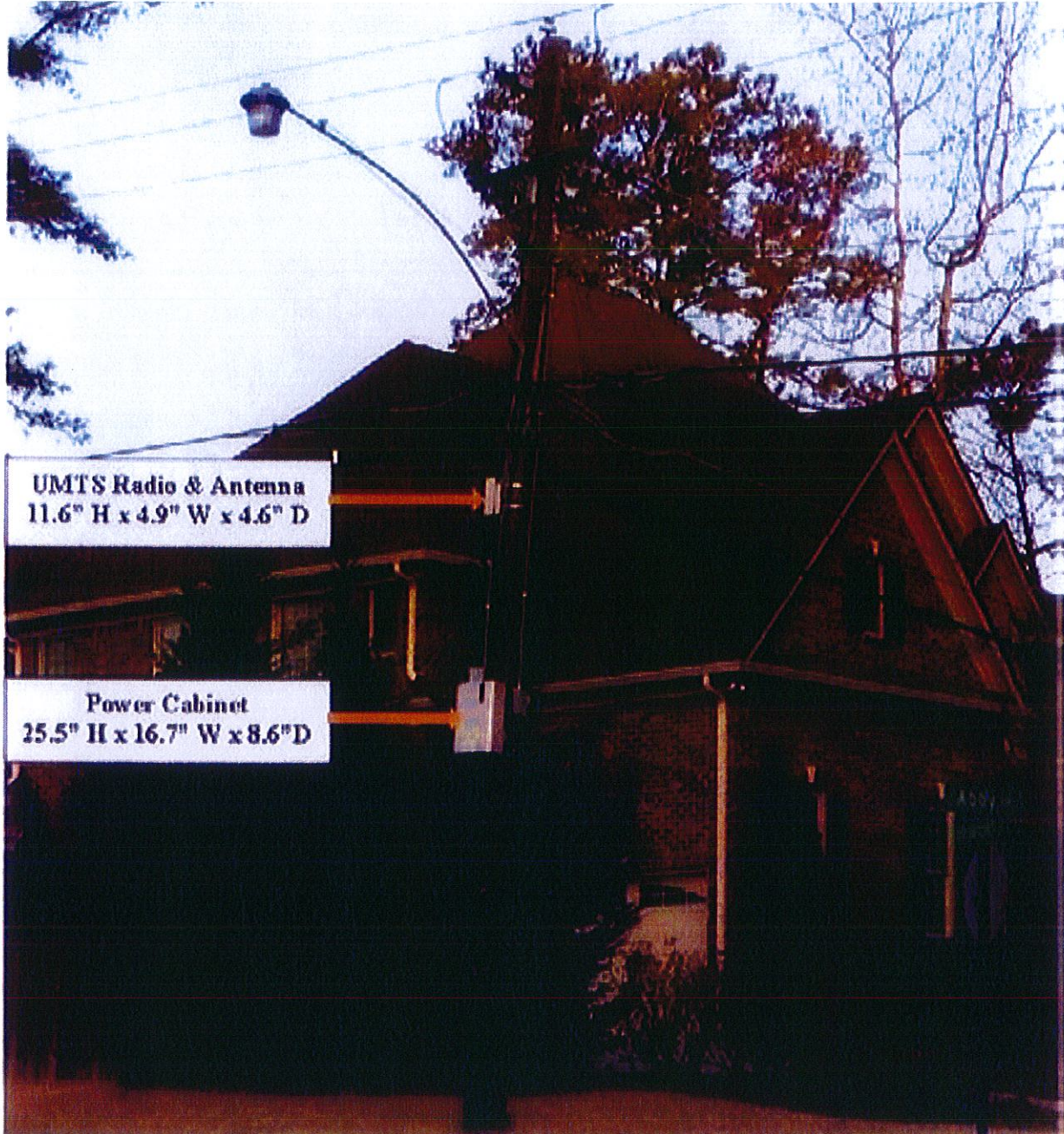
Figure 1. AT&T small cell deployment on a utility pole. 1
