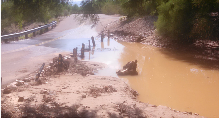
Fully charged drainage in Paradise Valley
