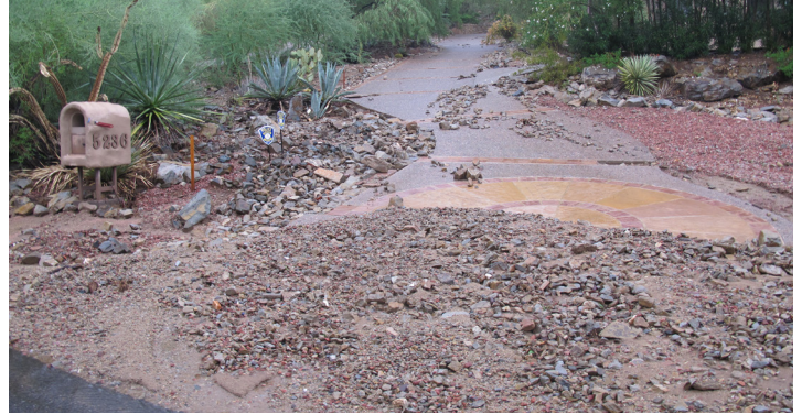
Erosion in Paradise Valley
