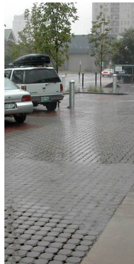
Permeable paving is an attractive way to provide runoff reduction in paving and pedestrian areas.
