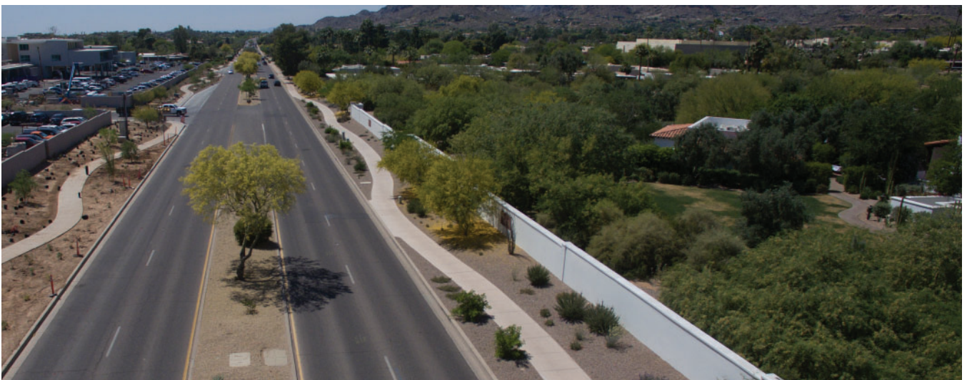
Figure 4.1: Landscape, Sidewalk, and Oleander Hedge Replacement Improvements on Lincoln Drive Completed in 2015
