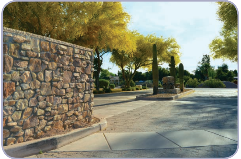
Figure 2.19: Example Use of Stone Veneer and Decorative Paving at Resort Setting
