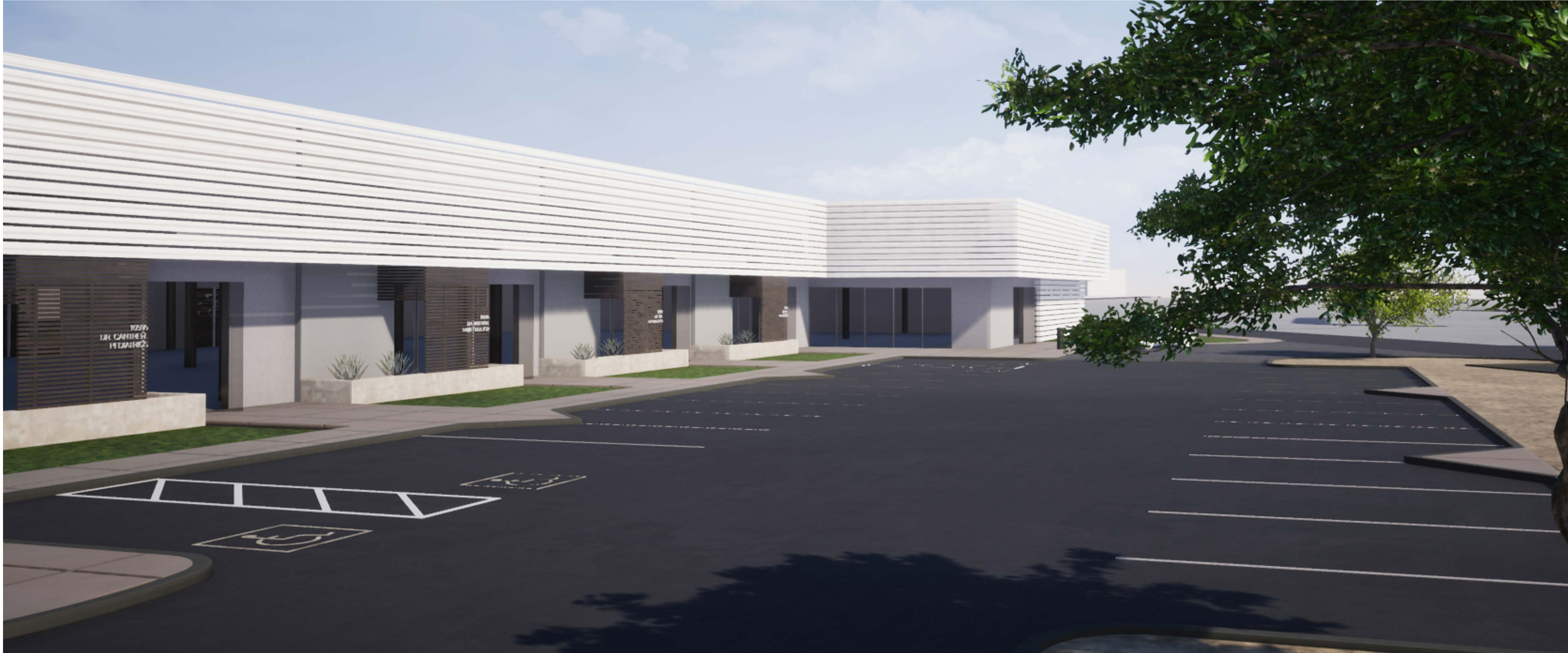
VIEW OF BUILDING F
