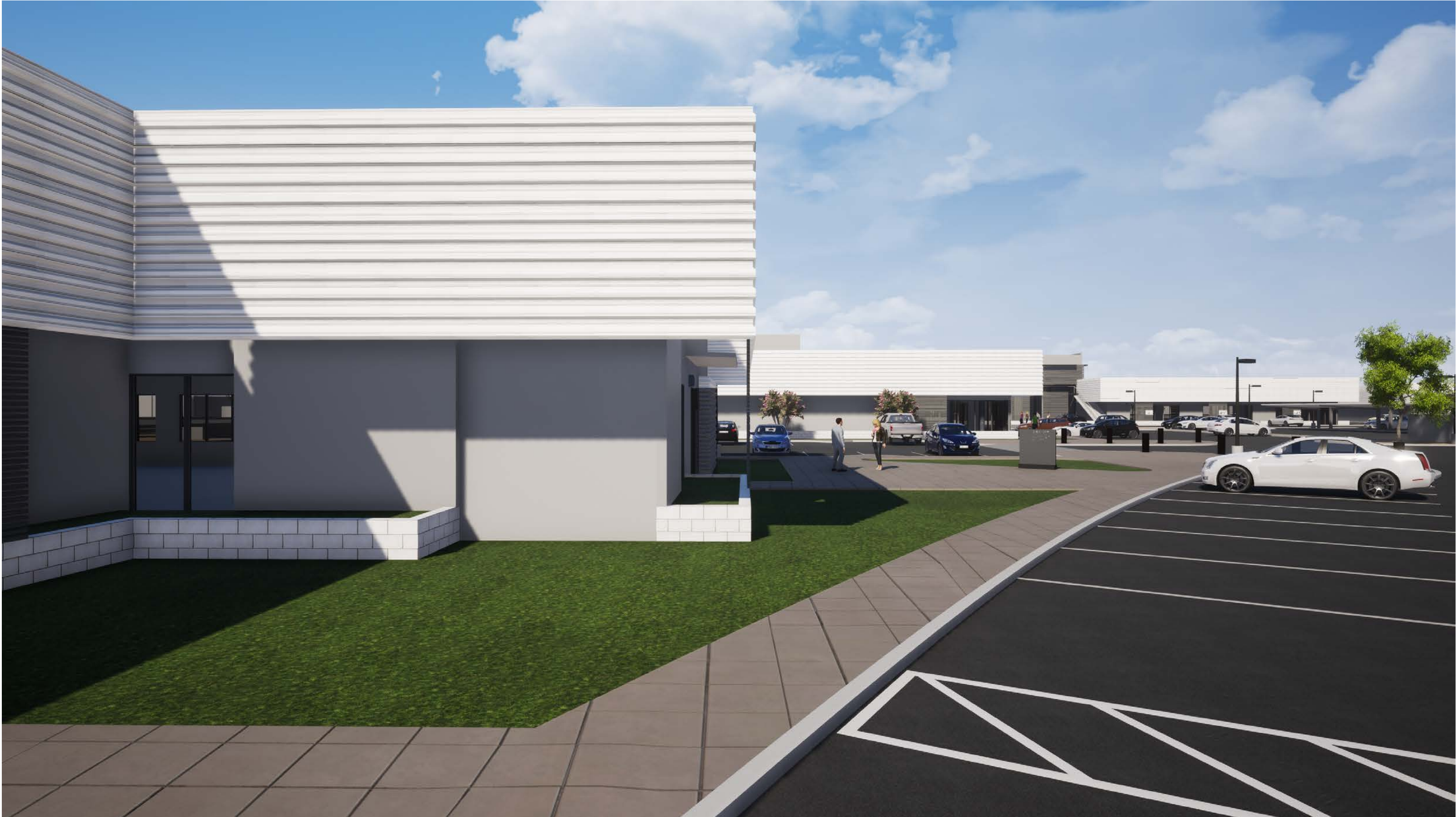
VIEW OF BLDG A LOOKING NORTH
