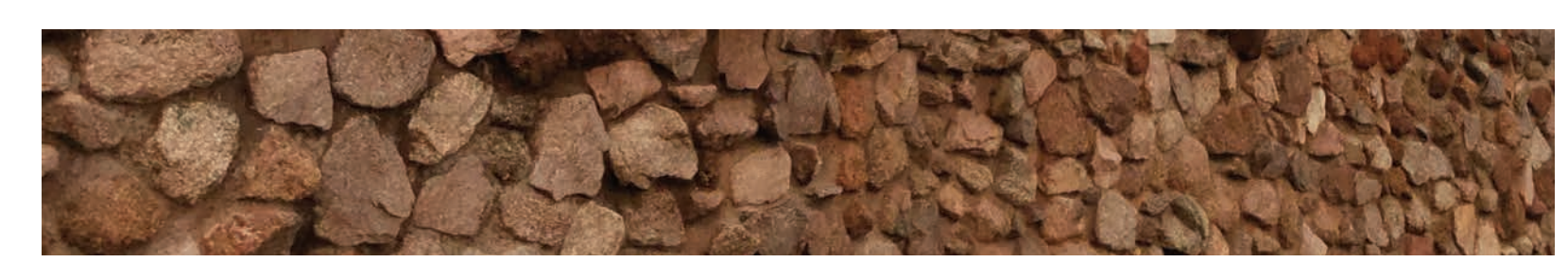
EXISTING STONE WALL LRV 11
